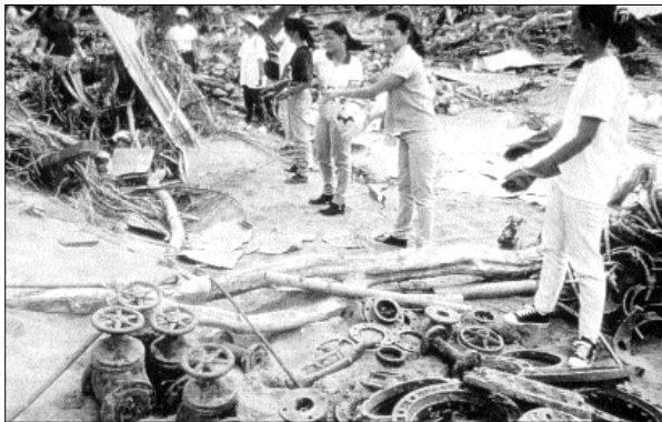
Damage to a water company's storage facility in Tegucigalpa, Honduras, following Hurricane Mitch.
