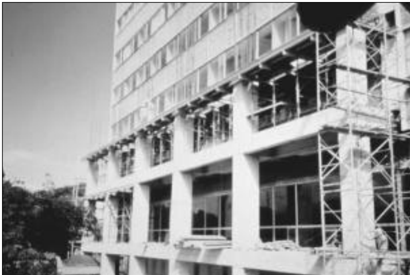
Photograph 14. Use of external perimetric frames for reinforcement of the Hospital Mexico in a project carried out by the Costa Rican Social Security Fund (CCSS).
