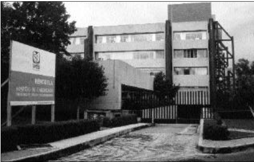
Photograph 12. The Cardiology Hospital of the Mexican Social Security Institute was retrofitted using buttresses following the 1985 Mexico City earthquake.
