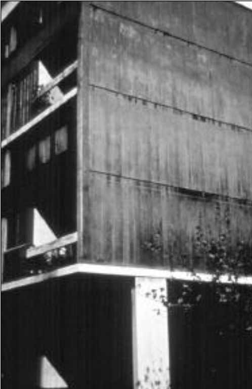
Photograph 10. Interruption of a structural wall on the ground floor
