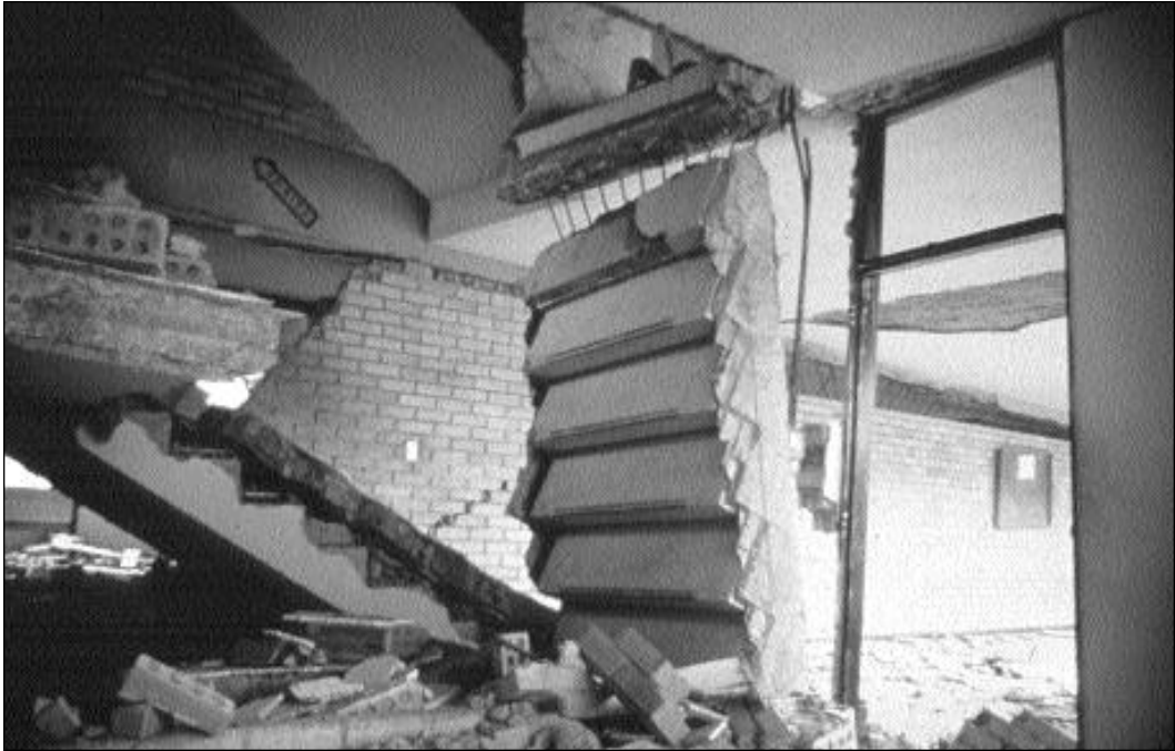
Photograph 6. Collapse of stairway during earthquake prevents evacuation.
