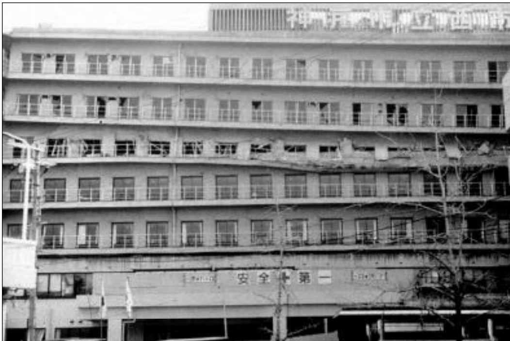
Photograph 3. Collapse of the fifth floor of the Municipal Hospital, Kobe, 1995.
