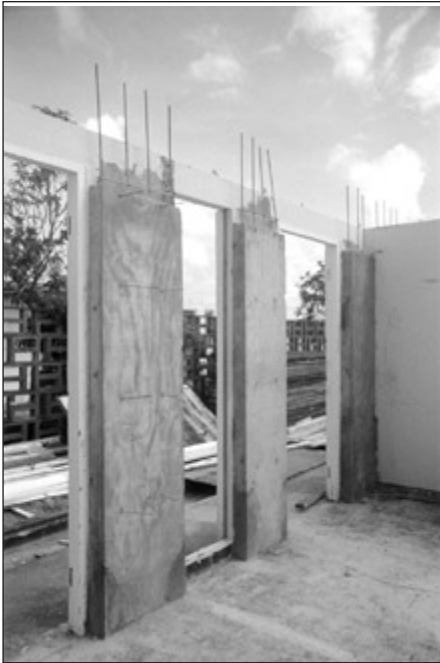
The strengthening of unreinforced masonry walls by applying a reinforced-concrete skin during the retrofitting of a hospital after hurricane damage. (Photo Tony Gibbs)
