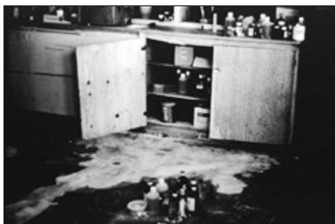
To reduce the losses and dangers from spilt chemicals and drugs, shelves and cupboards should be designed with adequate restraints. (Photo PAHO)
