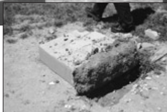
The absence of anchorage led to the removal and overturning of the entire building of this clinic in a hurricane. (Photo Tony Gibbs)
