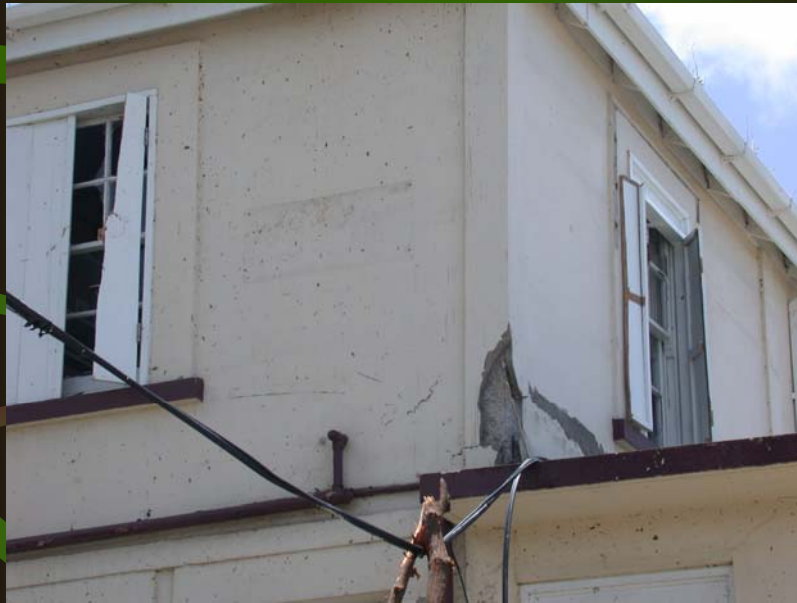
The Duncan Ward retrofit shutters broke
