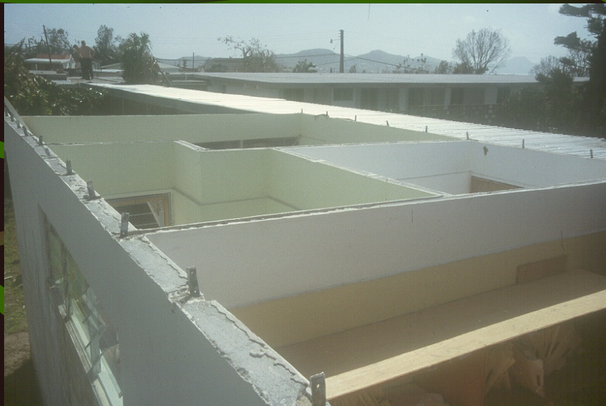
Structure lost in spite of clips
