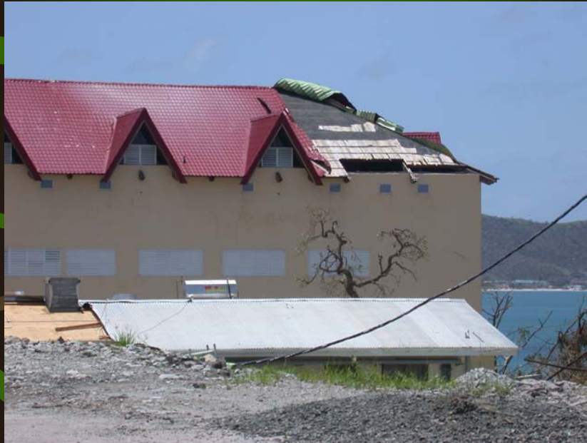
The New Hospital – Roofing Damage
