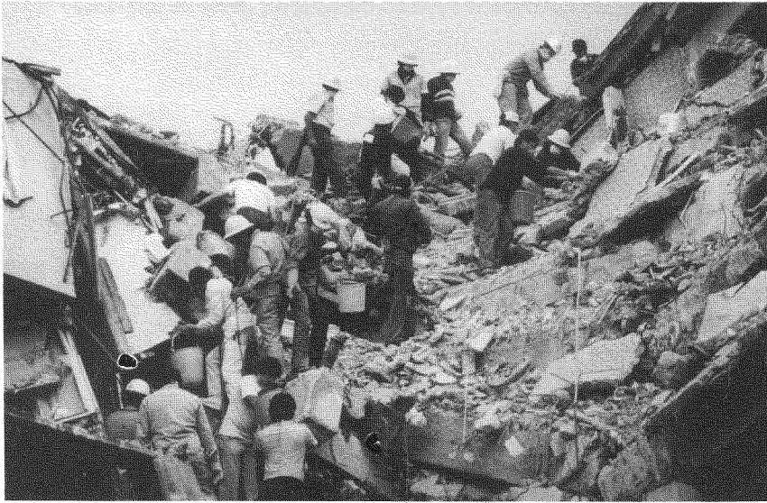
Fig. 18.5. Over 500 patients and health personnel were buried under the ruins of the Hospital Juarez in the Mexican earthquake of September 1985.
